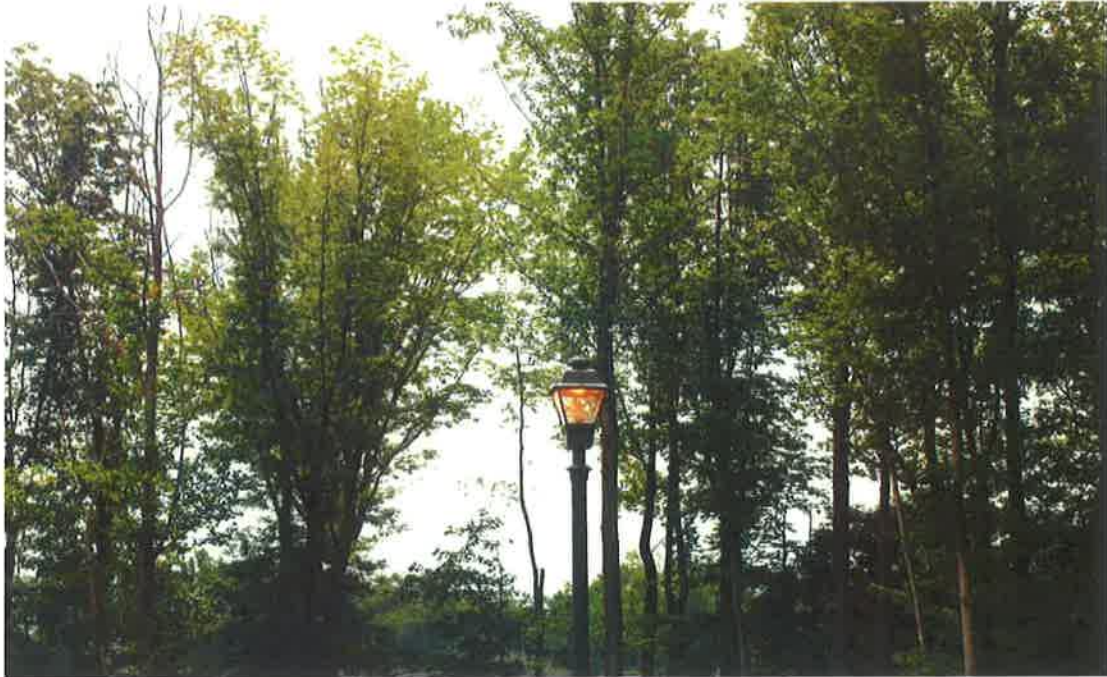
A pole light in the parking lot at Ryder Cup pool stays on all the time, likely due to a bad photocell.
