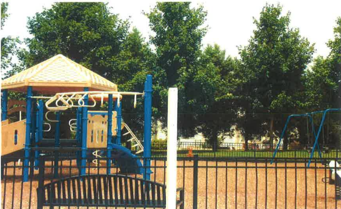
Missing sign at Waverly Park tot lot.
